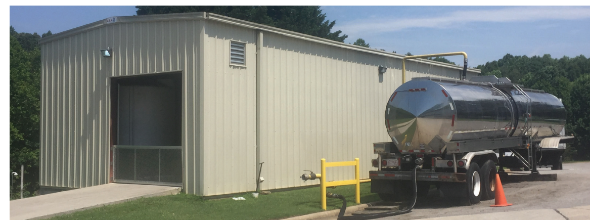
Reidsville Production Plant wastewater pre-treatment facility
