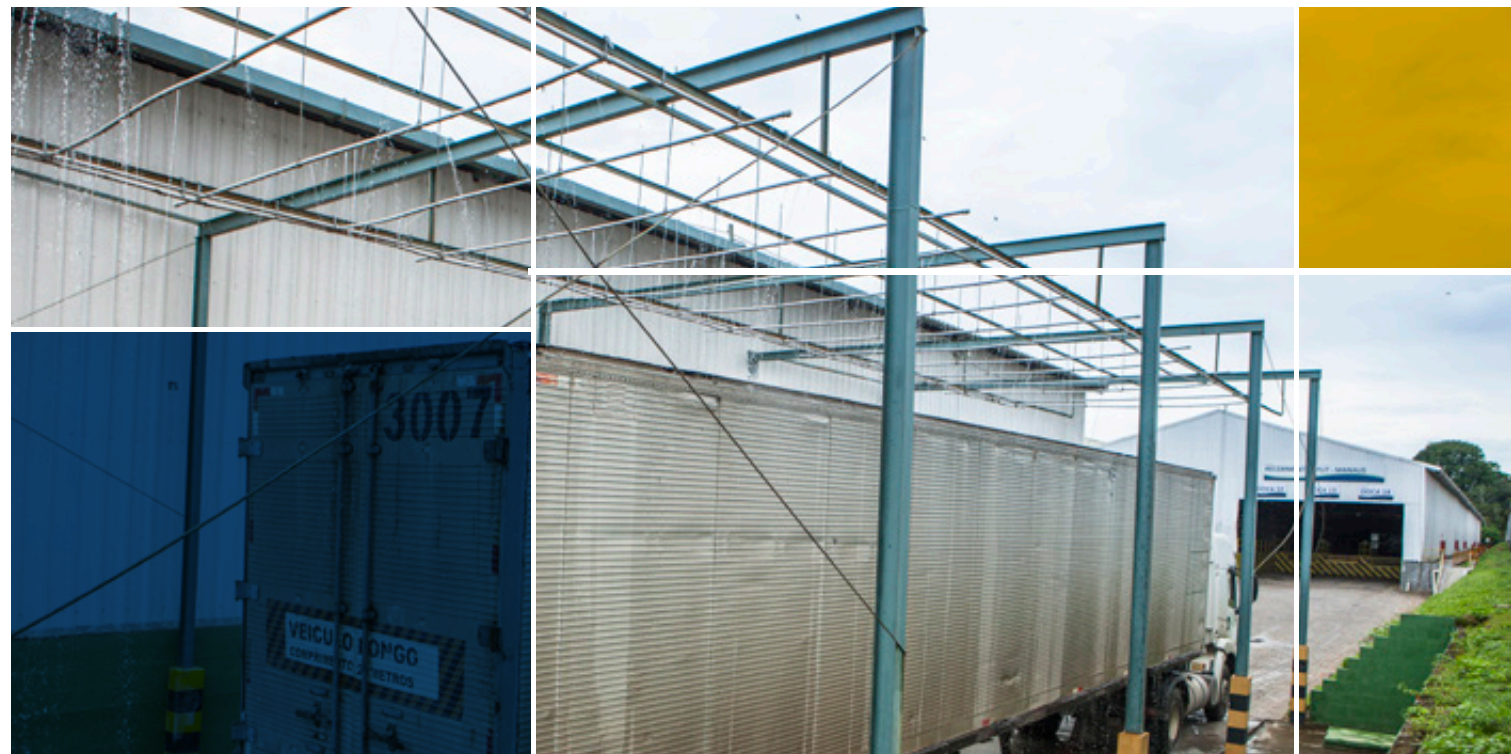
Rainwater reuse at the Manaus Unit, a process that identifies whether the vehicles carrying the products are free of leaks.
