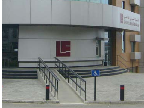
To facilitate access to its branches and its ATMs by persons with disabilities, BLF takes necessary steps to install ramps at selected branches.
