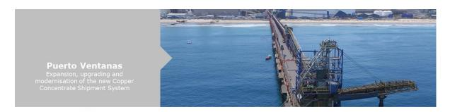
In the Puerto Ventanas Project, a belt system inside an enclosed gallery was proposed to the customer to prevent the emission of dust particles to the environment, in addition to scrubber systems at points with a risk of dust emissions.
