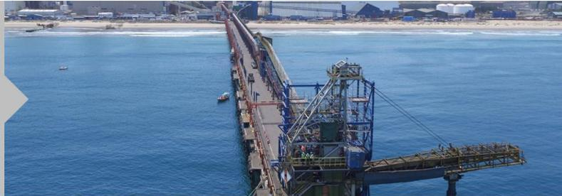
In the Puerto Ventanas Project, a belt system inside an enclosed gallery was proposed to the customer to prevent the emission of dust particles to the environment, in addition to scrubber systems at points with a risk of dust emissions.
