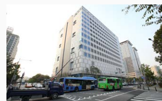
Mokdong IDC Center 2
