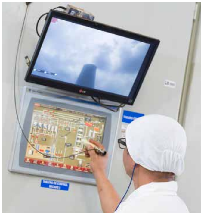
Emissions control system in the soluble coffee process, Colcafé Medellín.
