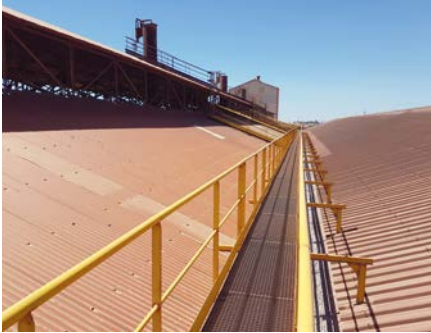
Safe access to roof
