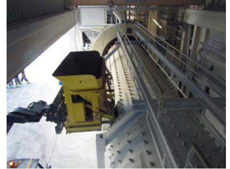
Grinding media being loaded into the mill
