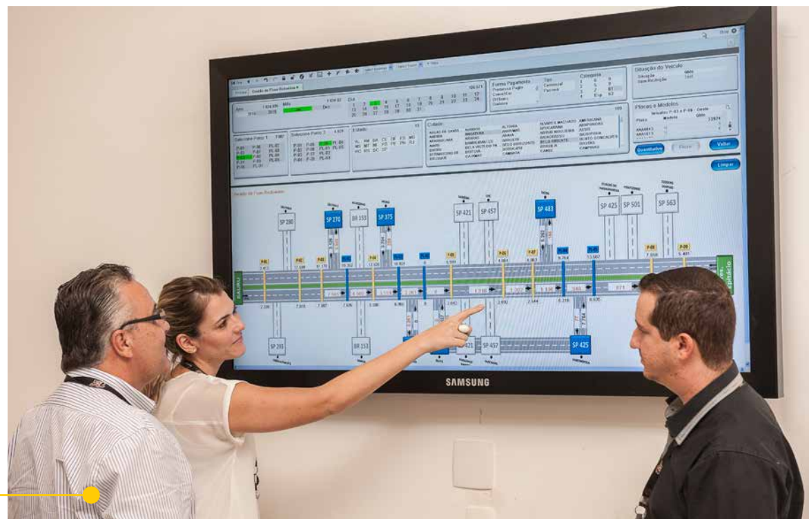
Painel de controle CART
