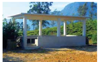
Resting Facility for Field Employees- Mattakelle Estate
