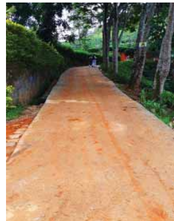
Road Concreting- Bearwell Estates
