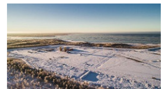
Hanhikivi 1 construction site.
