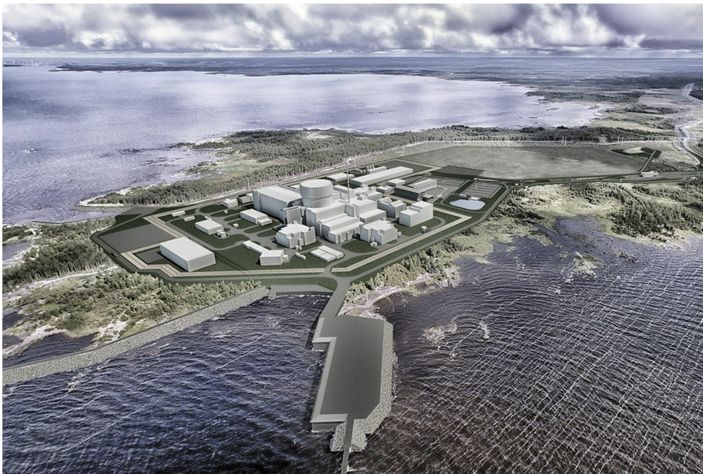
Hanhikivi 1 nuclear power plant: Photo: Fennovoima.
