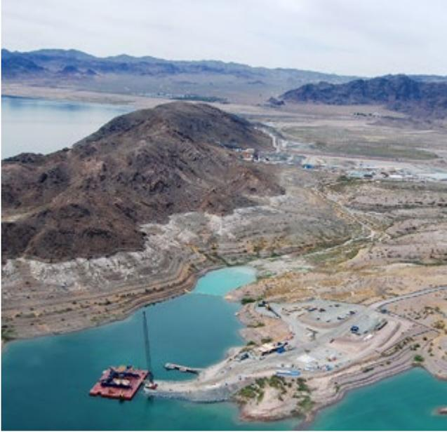
**Objective:** increasing the water supply for drinking and domestic use to the city of Las Vegas, through a complex underground system of collection and transport of water from Lake Mead
