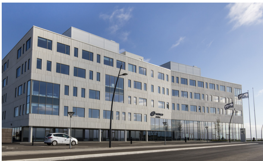
A sustainable new domicile with outstanding indoor climate, space efficiency and focus on low energy consumption.
