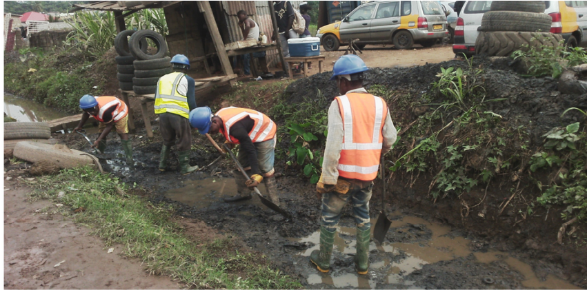
Plate 4.5: Desilting work in progress
