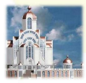
and successful trials with our rapid mould system. To bond the panels together Crystic BP 90-80PA was used. Altogether, we have supplied 70 tons of Fire-Retardant Resin and 5 tons of white fire-retardant gelcoat for this project. The end result is a very impressive looking church.
