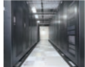
Disaster countermeasure center in the Kansai region
