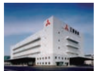
Sakurajima Warehouse No. 1, Osaka Branch
