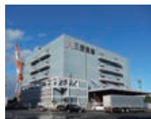
Daikoku Warehouse C, Yokohama Branch
