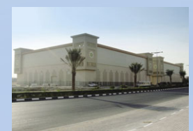
Discovery Garden DCS* Plant (Dubai) *DCS: District Cooling System
