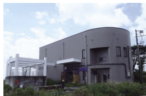
Disaster recovery construction of Yuriage rainwater pump station in Natori City, Miyagi Prefecture
