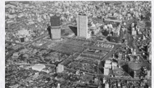
Shinjuku Fukutoshin District (District Heating and Cooling Systems)
