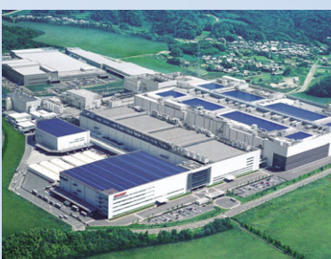
Sharp Corporation Kameyama Factory (Kameyama City, Mie Prefecture)
