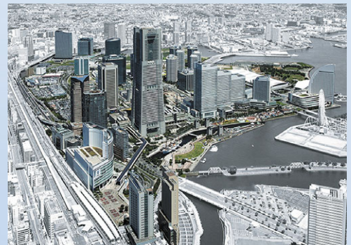
Minato Mirai 21 Central District DHC (Yokohama City, Kanagawa Prefecture)
