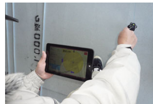
Marking using a tablet computer for installation operations
