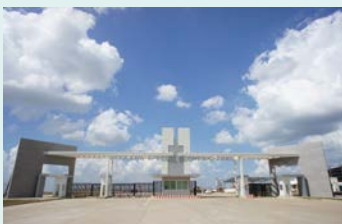
Main gate A of the Thilawa Special Economic Zone
