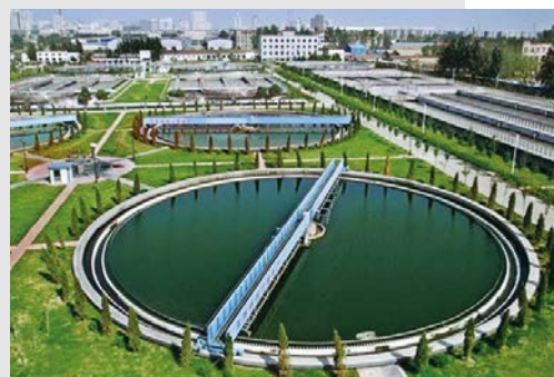
The sewage treatment plant in Linyi, Shandong
