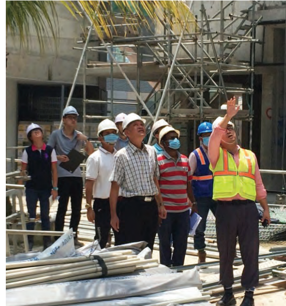
Workplace safety at construction site
