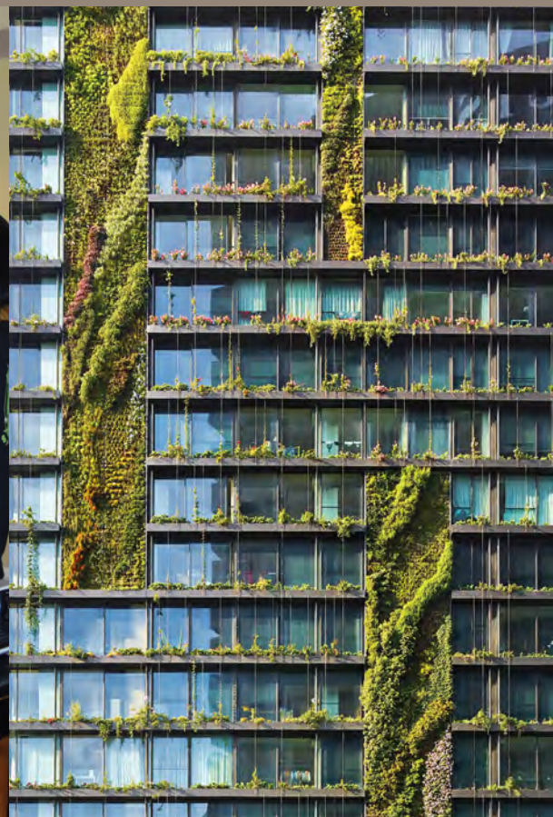
Vertical greenery at One Central Park, Sydney, Australia
