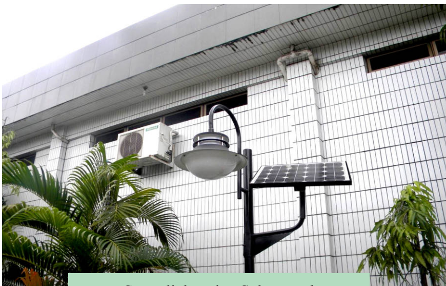
Street light using Solar panel
