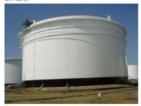
By keeping the temperature down, ZEFFLE helps prevent the transpiration of oil vapor inside the tank
