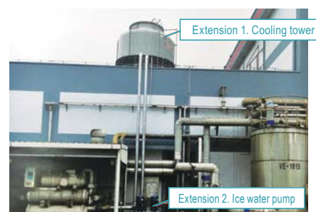
Upgraded cooling tower and water supply pump
