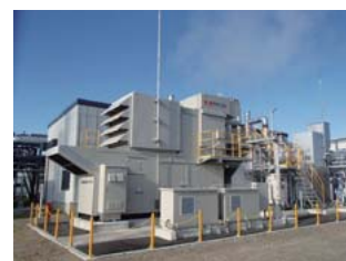
Natural gas turbine-powered cogeneration system at the Kashima Plant
