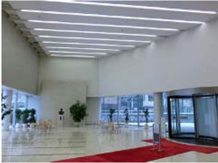
LED lighting in the lobby of the Hatsudai headquarters
