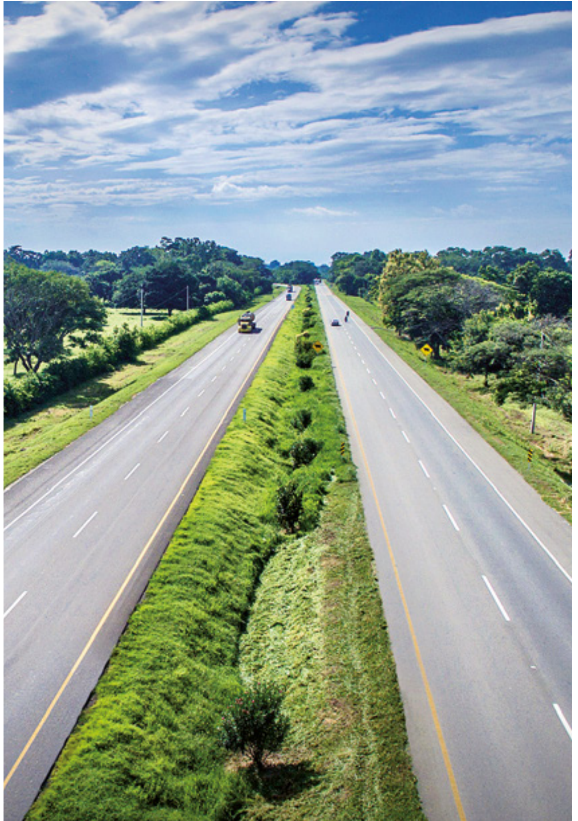
Over 1,000 km long, Ruta del Sol, in Colombia, is one of the most important highways in the country
