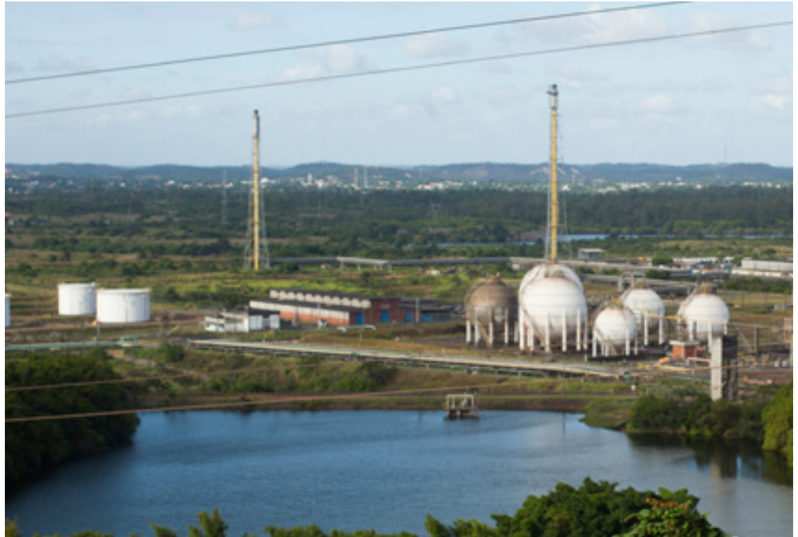
Reusing water at Unib 1, Braskem's main industrial plant at the Camaçari Complex
