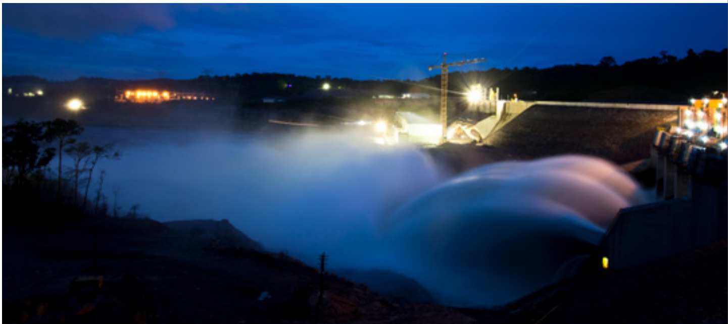
Teles Pires Hydroelectric Power Plant in Mato Grosso
