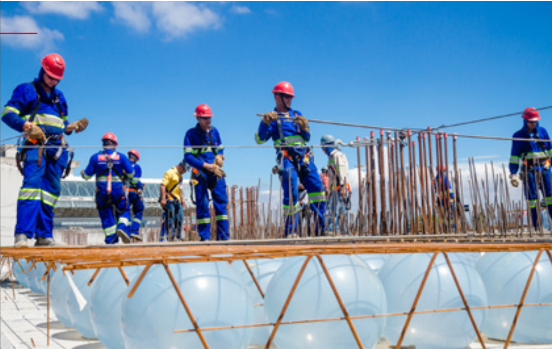
The Bubbledeck technology was used in slabs for the Federal District Administrative Center in Brasilia
