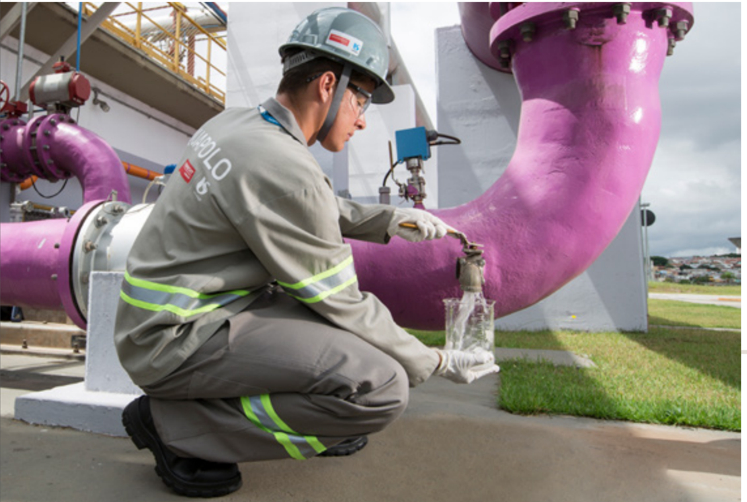
Member testing water quality: the company treats and supplies industrial reuse water to the ABC Petrochemical Complex in São Paulo State.
