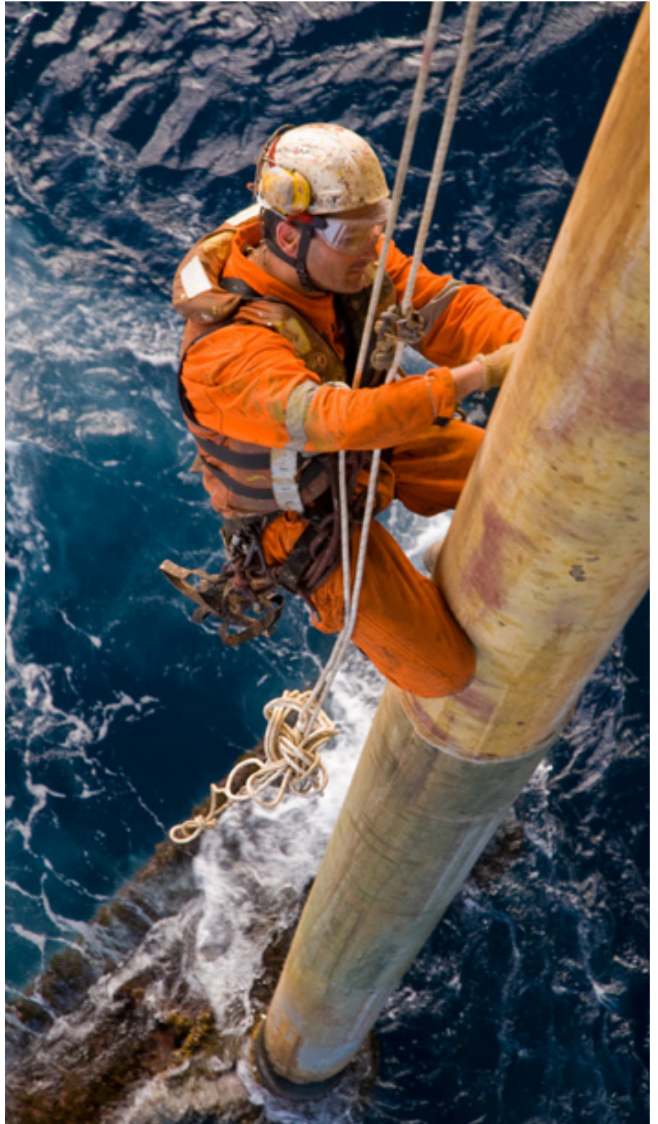
Odebrecht Oil & Gas Member doing maintenance work on an offshore platform
