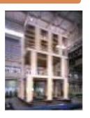
With renovation, Sumitomo Forestry offers its dual construction method for vibration control and seismic resistance (recipient of a Good Design Award in fiscal 2013), whereby the Sumirin REP construction method (the Company's original seismic resistance technology) is used to help to increase the seismic rating by at least 1.0.\*1 followed by the fitting of S-shaped vibration dampers.
