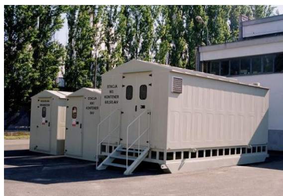
Containerized substations
