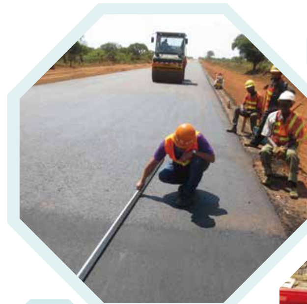
In the highway project in Zambia, Chinese employees are demonstrating how to measure the pavement levelness with a leveling instrument.
