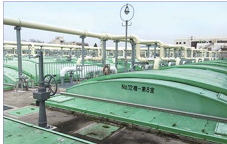
Project name Hirano Sewage Treatment Plant South Pond Reaction Tank Facility Project (Tank Nos. 7 to 12) Capacity Type: Diffusion plates in high-density configuration and low-power vertical stirring machine Capacity: 60,000 m³ per day Location Osaka Prefecture
