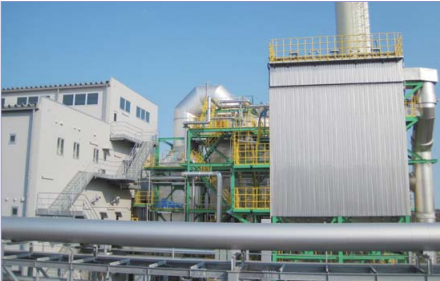
Project name Biomass Incineration Facility Installation Project Capacity Fuel: Paper waste Incineration capacity: 95 tons per day Location Fukushima Prefecture
