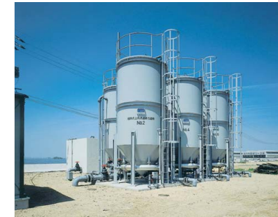
Upflow moving-bed filtration system
