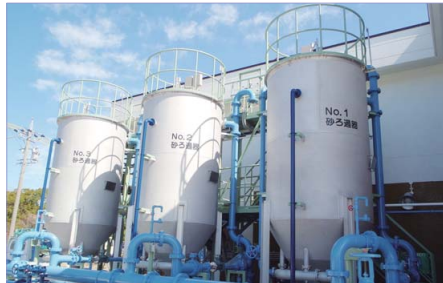
Project name Yokkaichi City Hinaga Sewage Treatment Plant Circuit 4 Water Treatment Facility Project No. 3 Project scope Disinfection facility, water supply facility, diversion manhole facility Principal systems Upflow fluidized bed filter M30UAG × 3 units Capacity: 1,800 m³ per day Location Mie Prefecture
