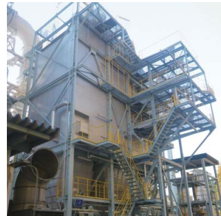
Waste heat boiler
