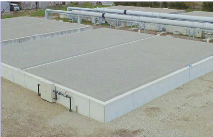
Project name Matsubara Preprocessing Plant No. 1 Soil Deodorization Floor Installation Project Capacity Type: Special soil, forced air Capacity: 85 m³ per minute Location Hyogo Prefecture
