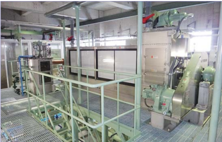
Project name Urado Bay Eastern Basin Sewage Treatment Plant Sludge Treatment Facility Project No. 10 Capacity Type: Pressurized screw press dehydrator Capacity: 24.2 m³ per hour Location Kochi Prefecture
