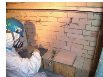
Repairing an incinerator's refractory
