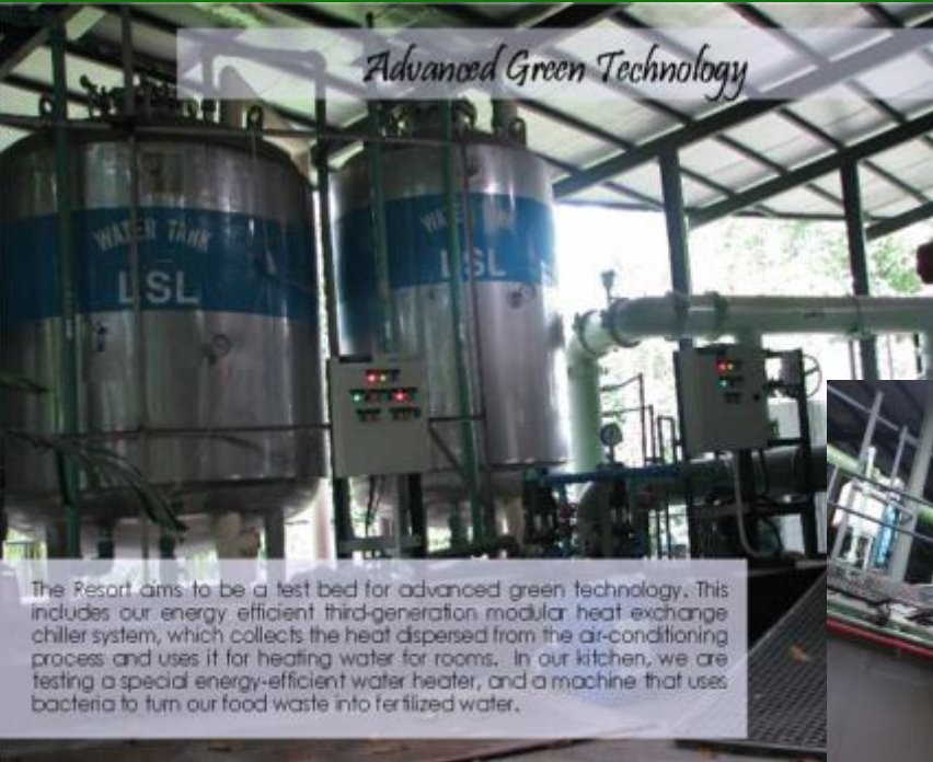
4 th generation modular heat exchange chiller system.
