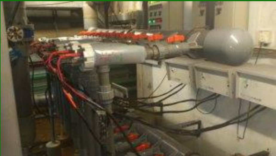
Swimming pool ionization treatment systems
