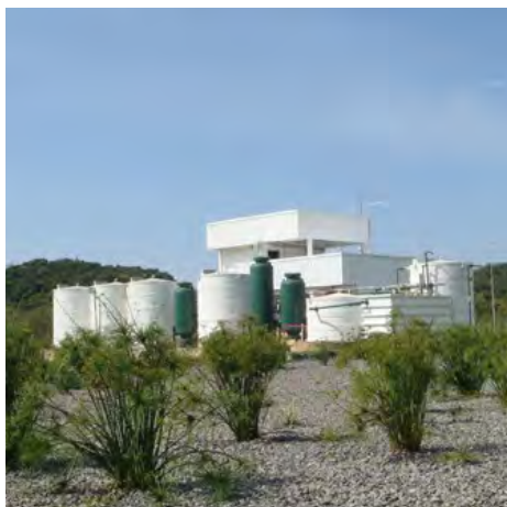
In Brazil, a wastewater treatment facility sits near Joinville Engine's filtering gardens.
