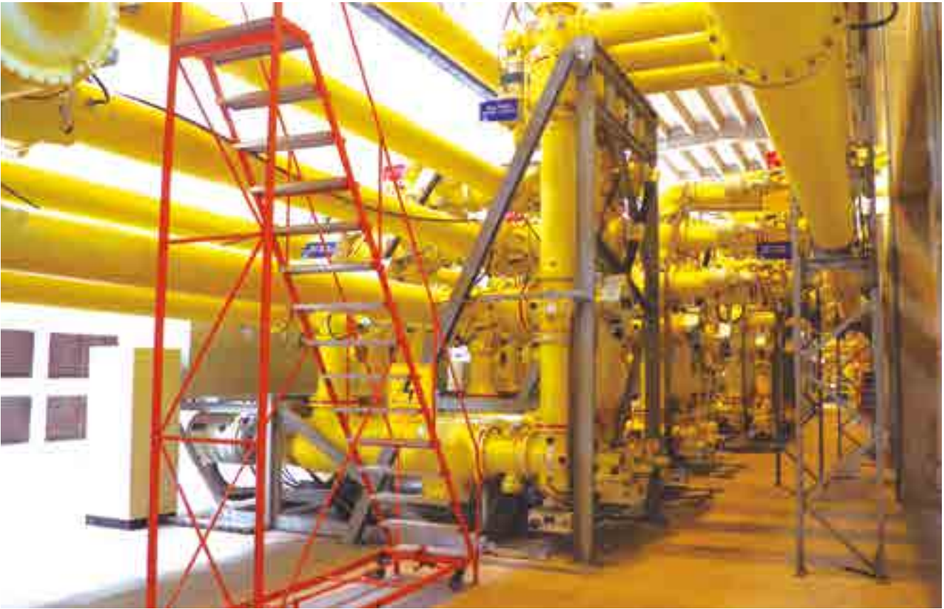
Photo 3. GIS Room of the Guavio electrical substation operated by EEB.
