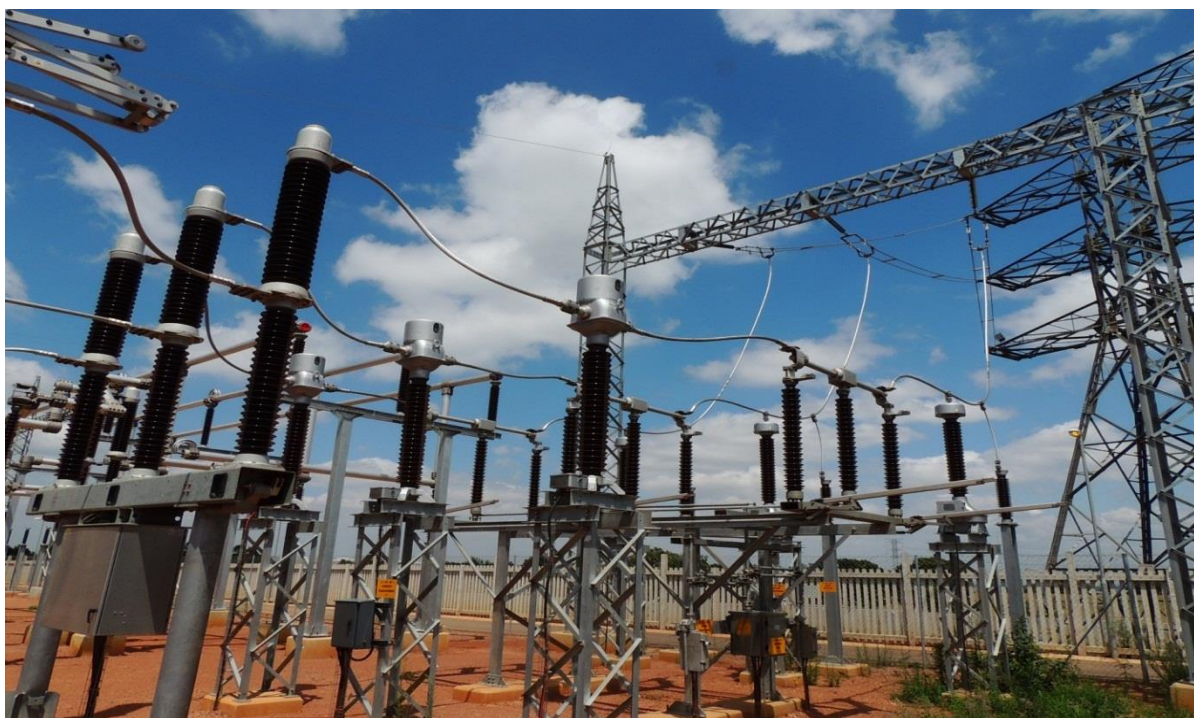
Figure 30: Rietvlei in-feed station (line in-coming bay)
