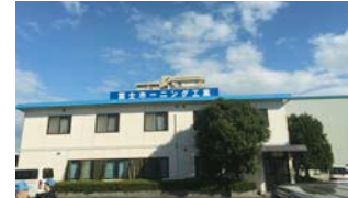
Fuji Honing Industrial currently has a BCP in place
