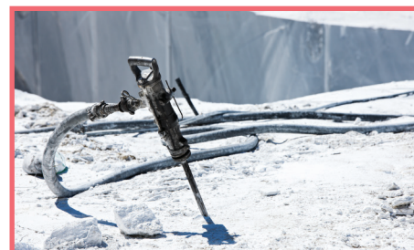
Preparing for extraction of natural stone
