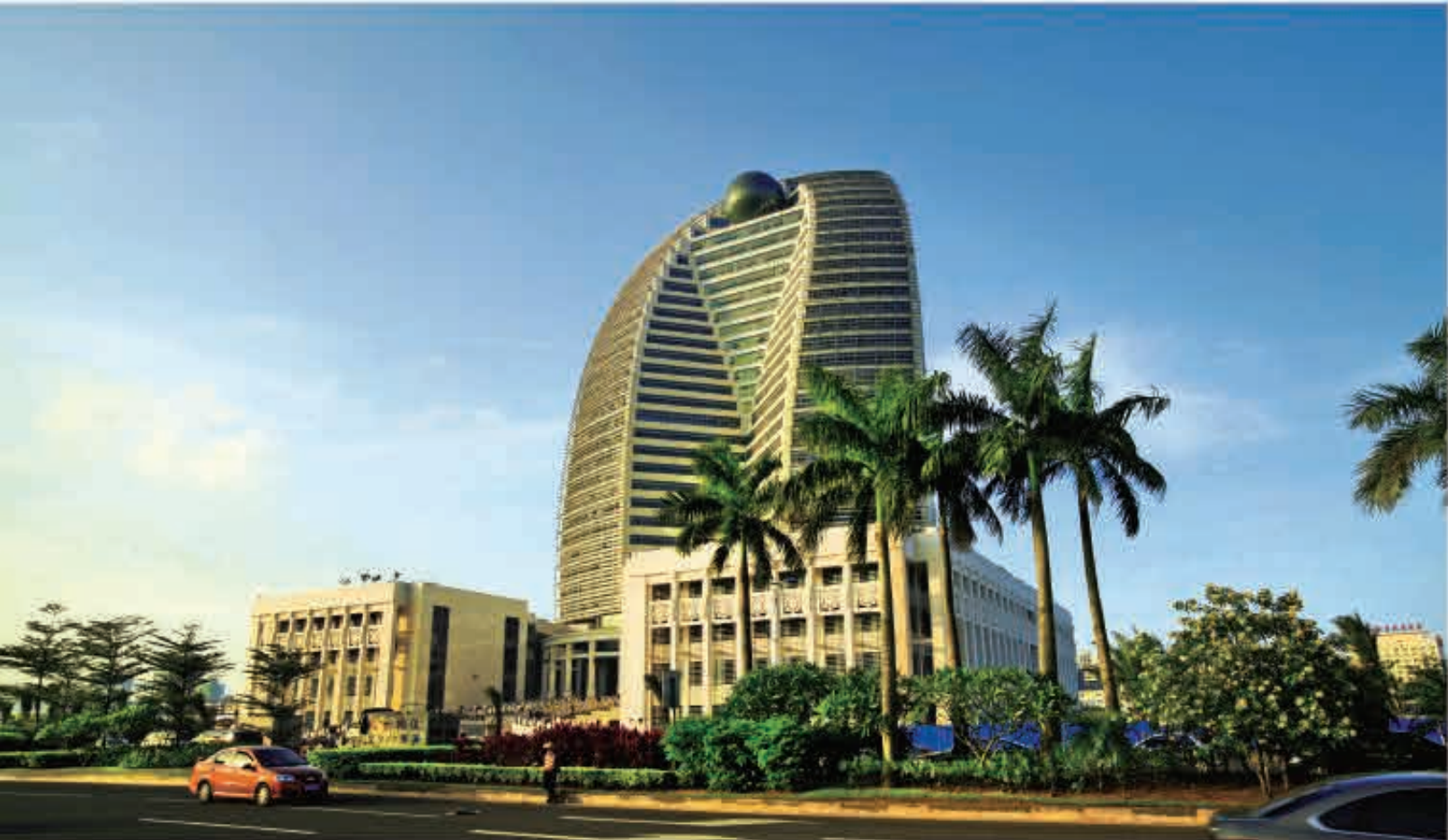
HNA Building in Haikou, China
