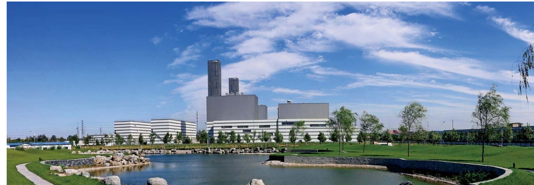
Beijing Cogeneration Power Plant
