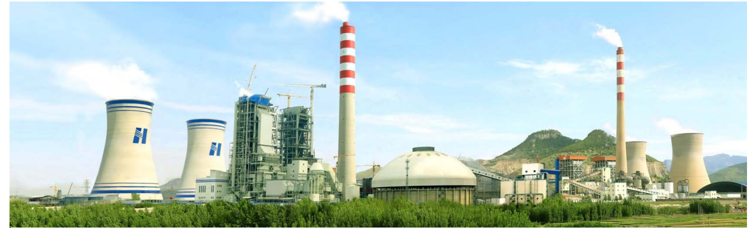
The first 1,000MW class ultra-supercritical double reheat unit of the Company and Shandong Province was put into operation in Laiwu Power Plant.
