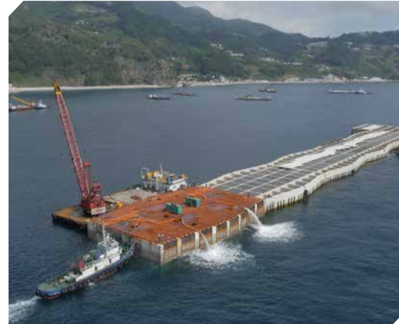
Floating breakwater construction site in Sadong port, Ulleungdo
