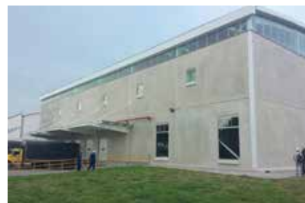
Distribution center for the Pasta Business in Mosquera, Colombia.
