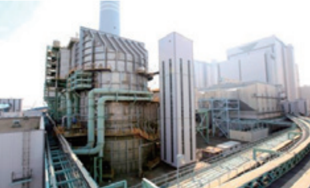
Yeongheung thermal power plant's Air Quality Control System (AQCS)
