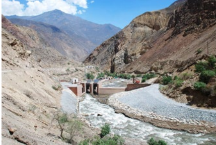
Bank stabilisation measures above the Huauro dam ahead of operation.
