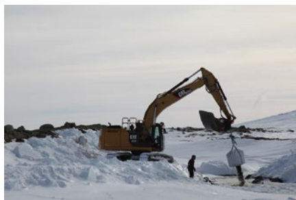
Djupa, Hardangervidda. Statkraft is adding gravel to the river bed to improve spawning conditions for the fish. Photo: Jon Aarbakk
