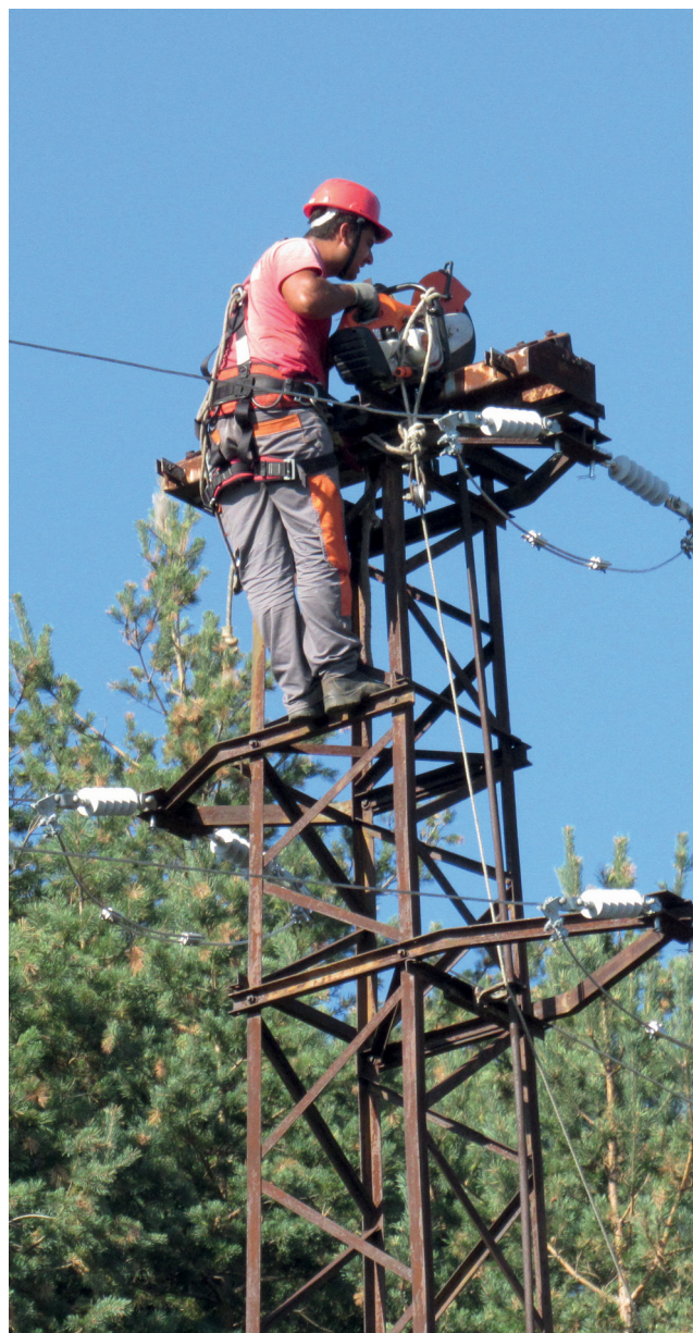
KEZ Kardzhali: repair of iron grid pillar on the overhead line at medium voltage "Ardino".
