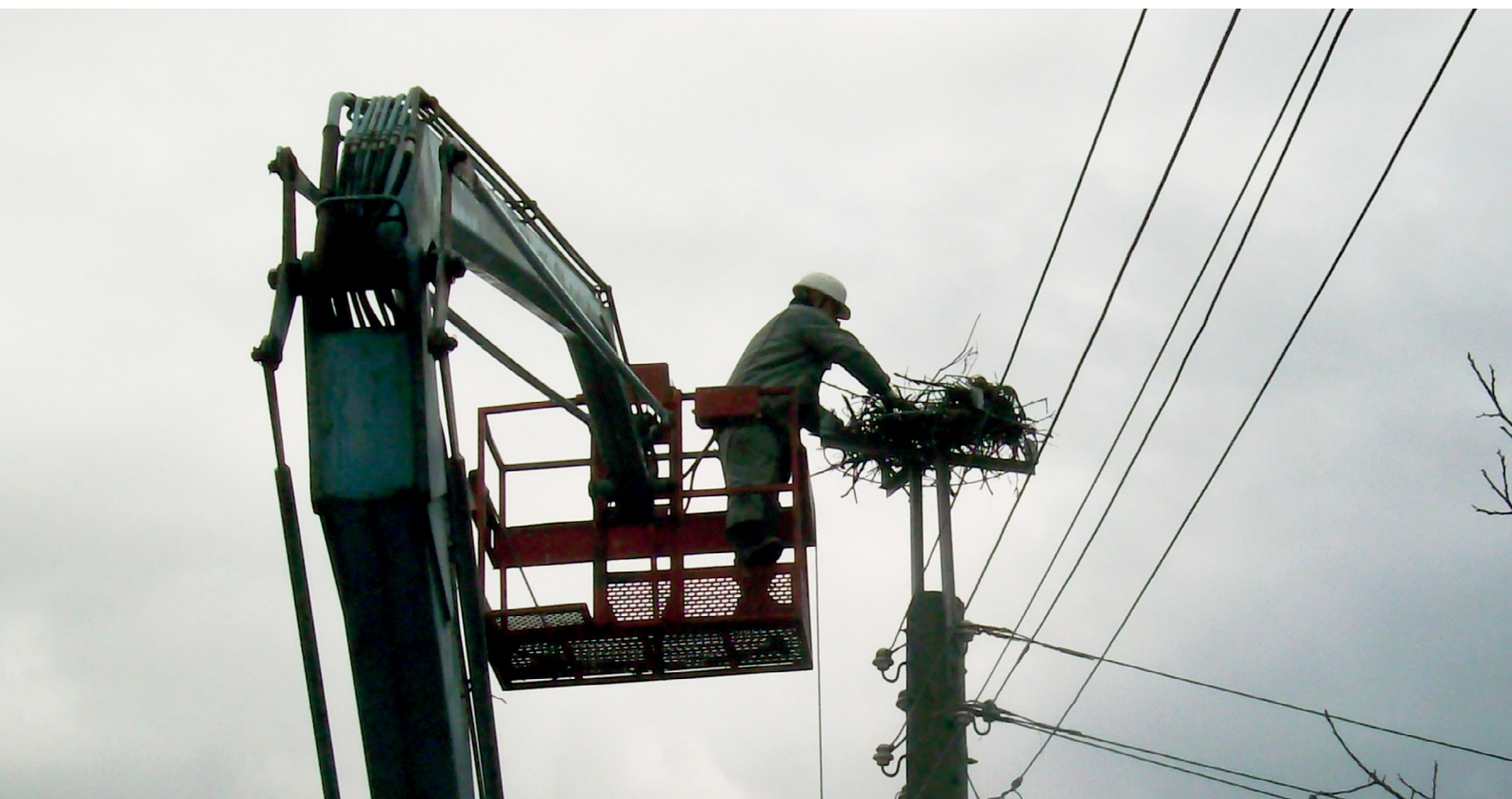
Installing the security platform for storks using the new and improved type in the region of Kardzhali.
