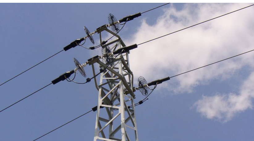
Insulators type "MST-spacers" were installed under the project "Life for Safe Grid".
