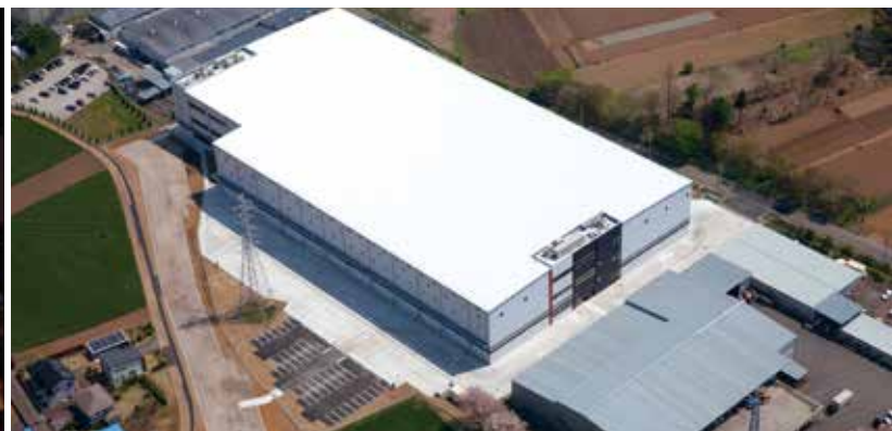
Moriya Logistics Center, developed in an ideal location for distribution (2016)
