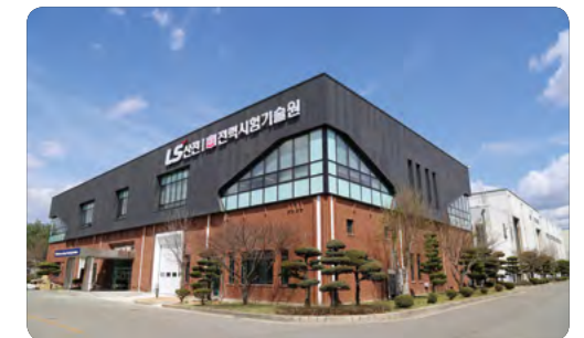
LSIS Power Testing & Technology (PT&T) Center
