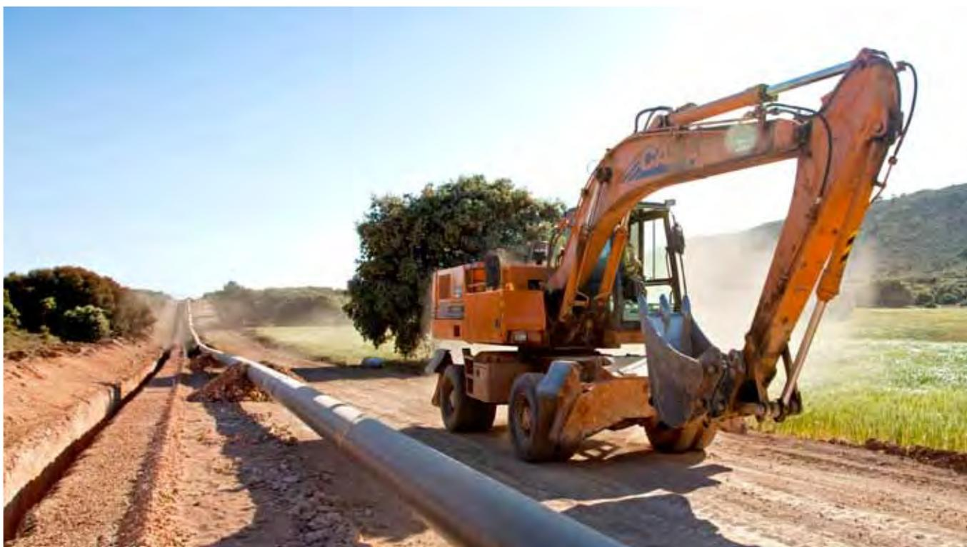
Anti-corrosion protection techniques used by the main gas pipeline operators worldwide are applied to all steel networks of Redexis Gas, whether gas pipelines or distribution branches. The application of such techniques as Integrity Management increases the useful life and notably reduces repairs, particularly corrective maintenance.
