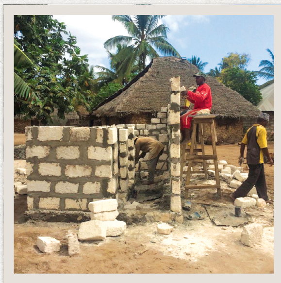
In 2015, the local seaweed farming community on Pemba Island, Zanzibar, Tanzania, was hit hard by a cholera outbreak due to poor sanitation infrastructure. Working with the Pemba Foundation, FMC financed the construction of public toilets to support healthier living conditions for the community. Photo Credit: Pemba Foundation
