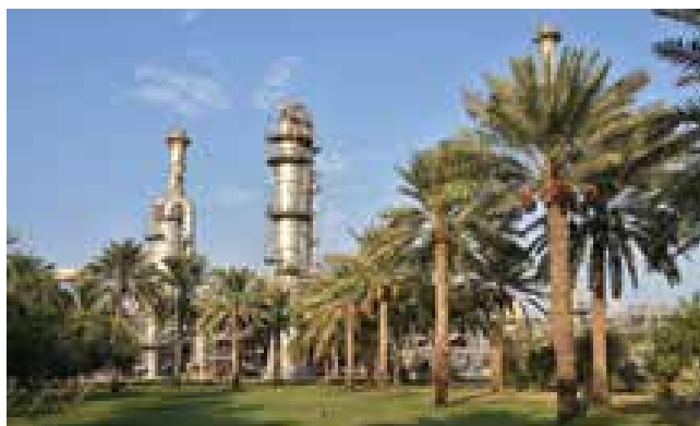
Operational excellence is our hallmark
