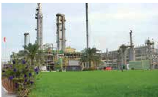
GPIC's Ammonia plant
