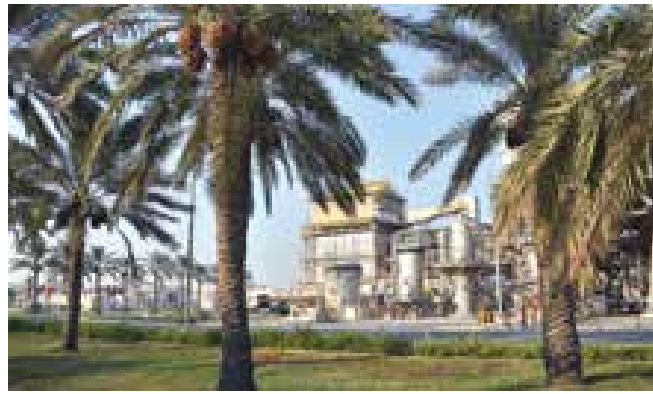
GPIC's methanol plant
