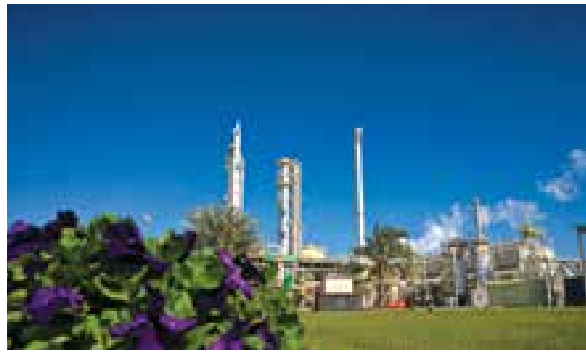
At GPIC, technology and nature co-exist
