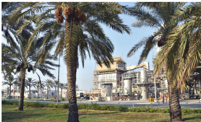
GPIC's methanol plant
