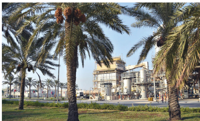
GPIC's methanol plant
