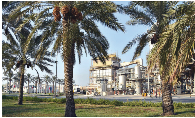
GPIC's methanol plant
