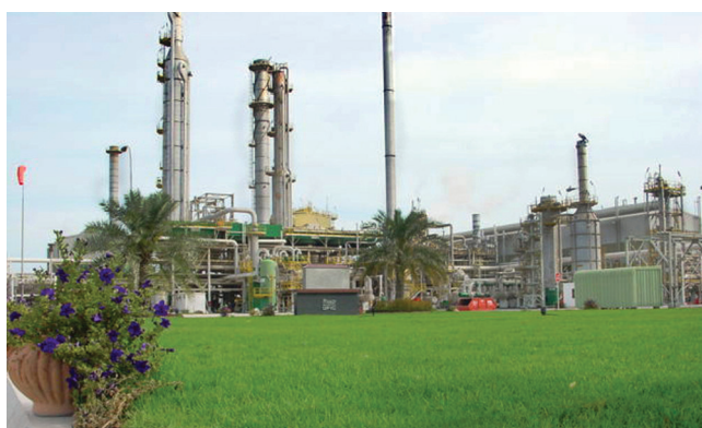
GPIC's Ammonia plant
