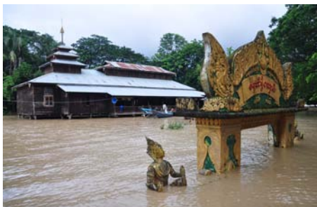
Flooding damage – Ayeyarwaddy Region (Danbi Township)
